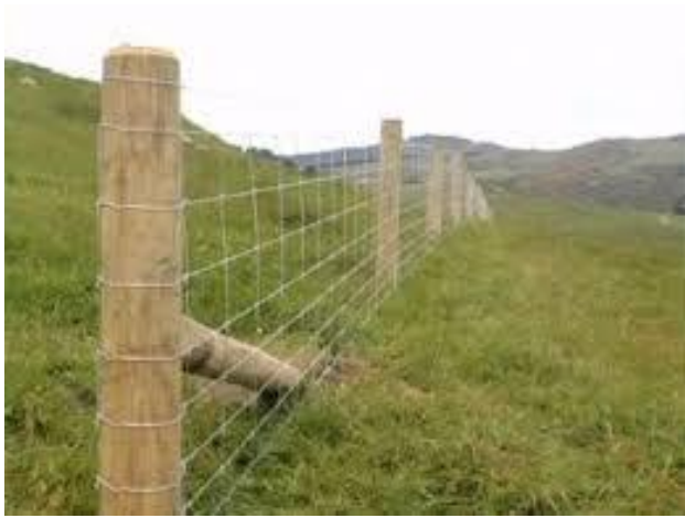
Fig.11 Sample woven wire perimeter fence for sheep and goat
