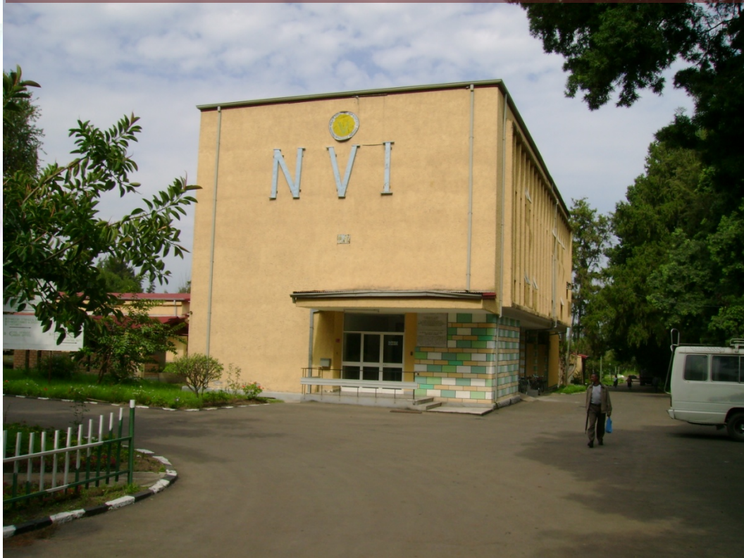
Figure 16: Front façade of the NVI
